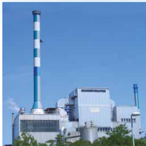
© Lühr Filter, Biomass Combustion plant. Reproduced with kind permission.
