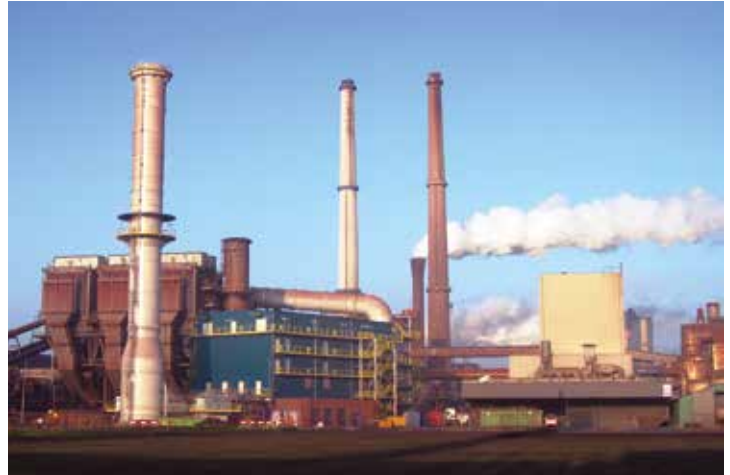
© Lühr Filter. Integrated Steel plant. Reproduced with kind permission.
